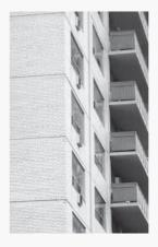
**Fig. 26.** Typical concrete slab with exposed slab edge and masonry facade
