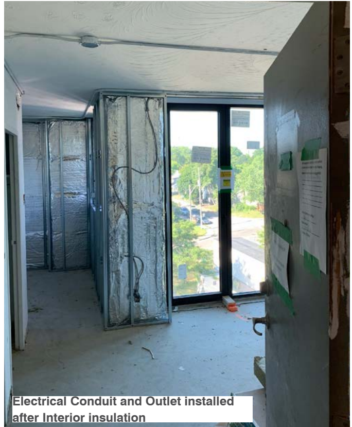
Exposed Conduit of Fire Alarm in Suite
