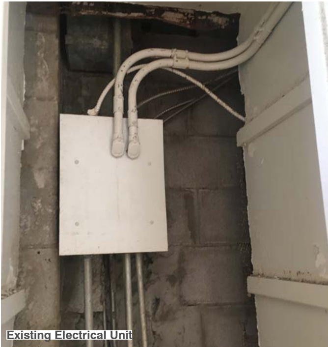
Exposed Conduit of Fire Alarm in Suite
